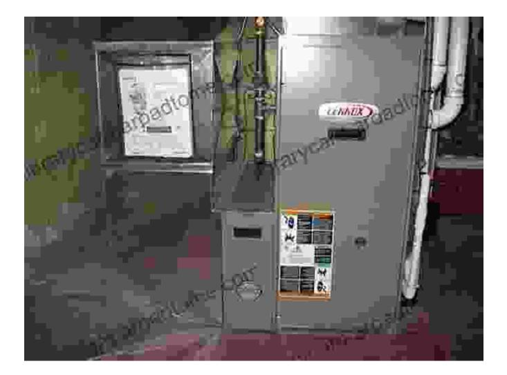
Furnaces reign supreme as the most prevalent home heating system, generating heat through combustion of fuels such as natural gas, propane, or oil. They distribute warm air throughout the house via a network of ducts, providing a reliable and efficient method for combating winter's chill.
